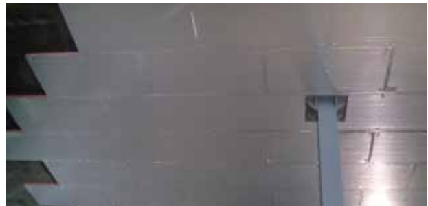
Figure 6 Board joints squared
