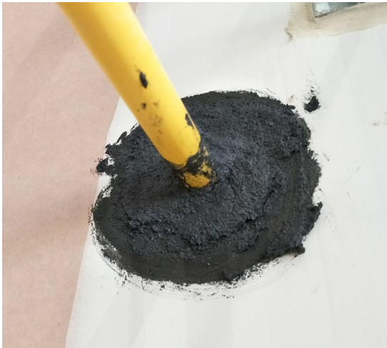
PEX-AL-PEX pipe and FYREPEX™ Sealant in a 2 hour plasterboard wall
