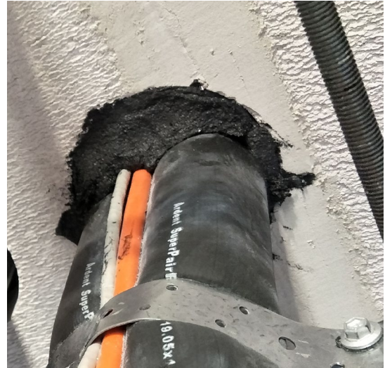
Mixed services treated with FYREPEX™ Sealant in a Hebel wall
